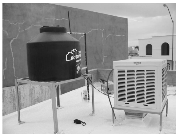
Figure 3: Evaporative cooling system
