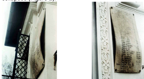
Figure 2: Bowing marble panel at a church, in Bucharest
