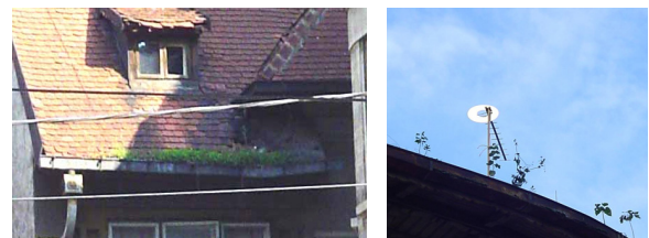
Figure 5: Poor maintenance helps vegetation grow on the utter
