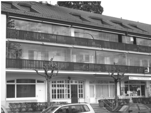
**Figure 11 :** Bellevue, Geneva, Sliding glass panels over balconies on a mid XX<sup>th</sup> century building.
