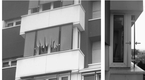
**Figure 5 :** Detail of a transformed balcony in a bow-windows and sight of solar protections in fabric torn.
