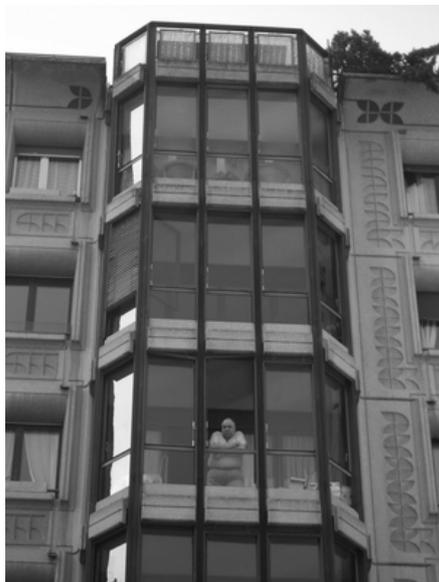
**Figure 4 :** Recently built housing block. The balconies were closed at the time of building. After 3 years of normal use, the first damage to the interior of the loggia due to condensation have appeared.
