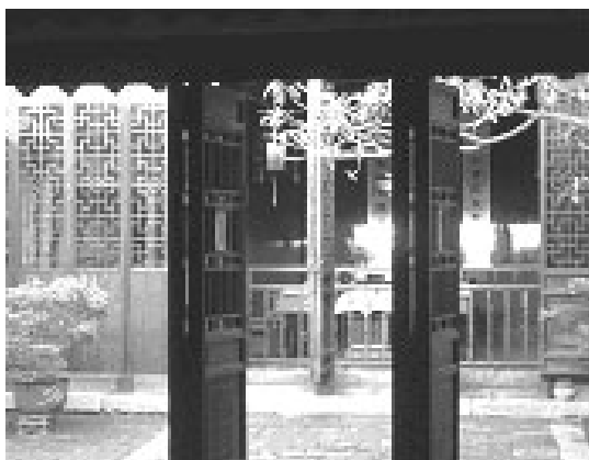
Figure 11: 'Crab Eye' light well acts as wind barrier, picture wall and ventilation shaft.
