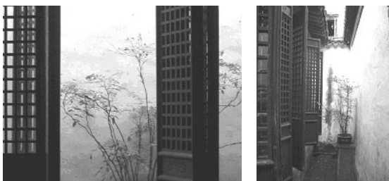
Figure 11: 'Crab Eye' light well acts as wind barrier, picture wall and ventilation shaft.
