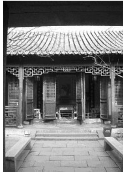
Figure 4: Roof of the ceremonial hall screens the sky to reduce glare in the eyes of the visitor
