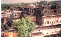
Figure 9: compact settlement allowing for mutual shading
