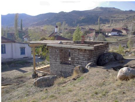
**Figure 3:** Building with mudbrick
