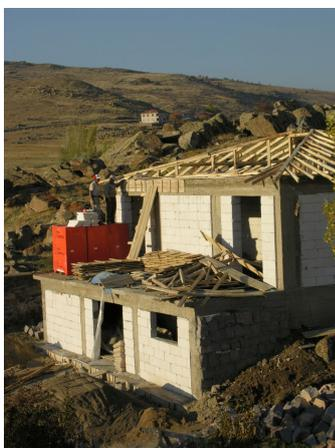
**Figure 5:** Building with Aerated Concrete and reinforced concrete frame
