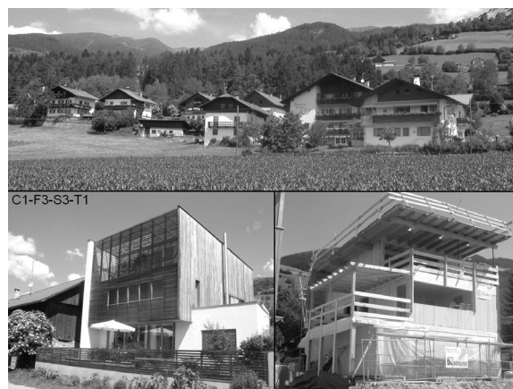
Figure 8: Wooden buildings at Issengo.
