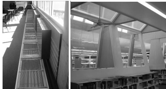
Figure 4: Photograph of; a) first floor air inlet louvres on the eastern side of the building. Note the early morning sun penetration, b) Clerestory above the library resource area. Note the ground floor flues are connected directly to outdoors to prevent short circuiting with the first floor.
