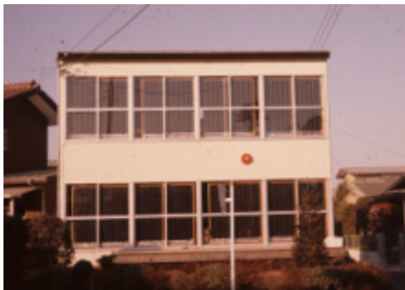
Figure 5: South side view of original K Solar House
