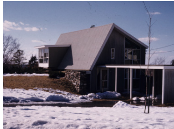
Figure 4: Outside view of the remodelled house
