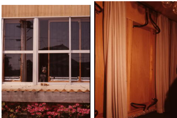
Figure 6: Collector of sliding doors partially opened (left) and inside view of them closed, where connecting rubber hoses can be seen (right)
