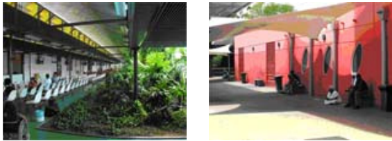
Figure 4. (left) Entrance to Sarah Kubitschek hospital. (right) Entrance to new wing, Royal Darwin Hospital.
