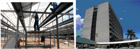
Figure 12. (left) Pre-fabricated lightweight construction system used at Sarah Hospital. Photo from Lele's archives (right) Royal Darwin hospital and its vertical concrete structure.
