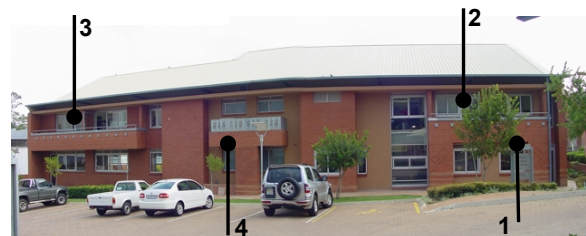
Figure 11: Northern façade of building showing the monitoring points
