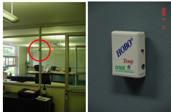
Figure 7: Monitor on mullion
