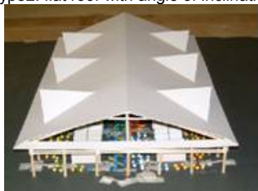
Type 3: pitched roof with openings
