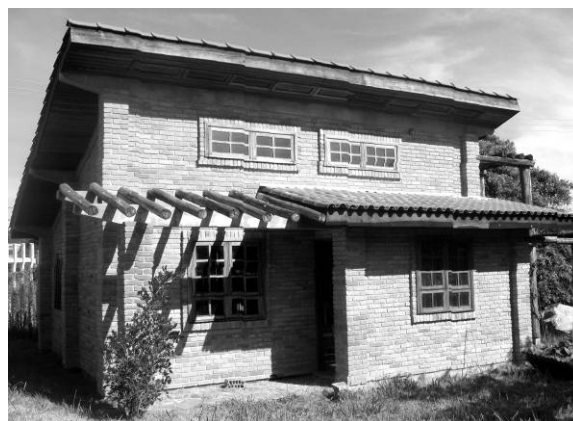
Figure 1: North façade of Alvorada Prototype
