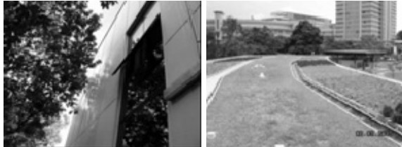
Figure 9: Measurements on building facade and rooftop (Left: tree-shaded façade; Right: rooftop garden).
