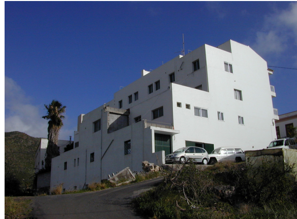
Figure 2: The museum storage is located on the lowest floor level where cars are parked along the side of the building. This is a view from the north.
