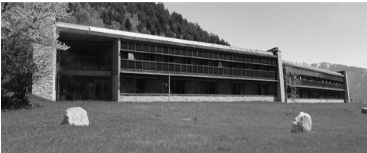
Figure1: Planes de Son, south façade
