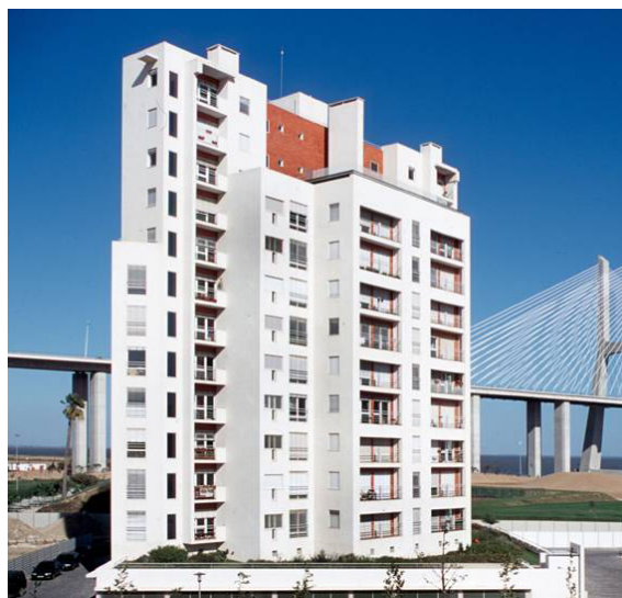
Figure 5: Passive solar building on the Expo98 site in Sevilla
