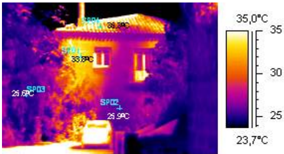
Figure 8: Thermographic view of the traditional house.
