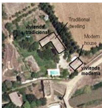
Figure 6: Aerial photo pointing out the location of both buildings.
