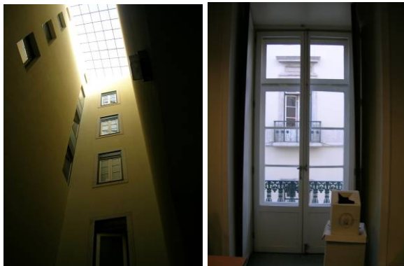
Figure 9: Skylights and window with an internal shutter
