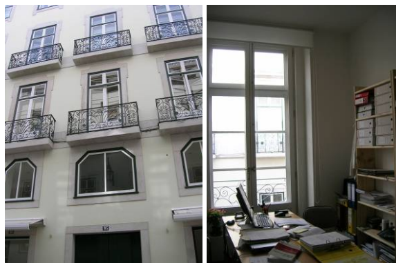
Figure 3: Castro and Melo Building
