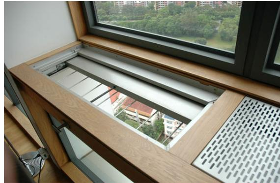
**Figure 6:** Monsoon window at One Moulmein Rise, Singapore, with slideable panel to regulate airflow.
