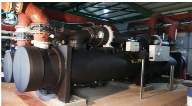
Figure 1: 10MW Centrifugal heat pump
