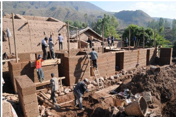
Figure 8: build a demonstration rammed earth house
