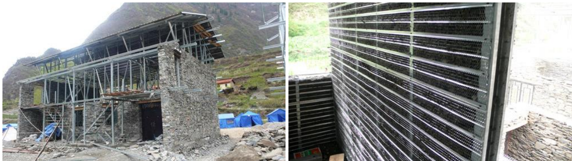
Figure 5: framework of reconstruction house Figure 6: a double-sided hot-dip galvanized network
