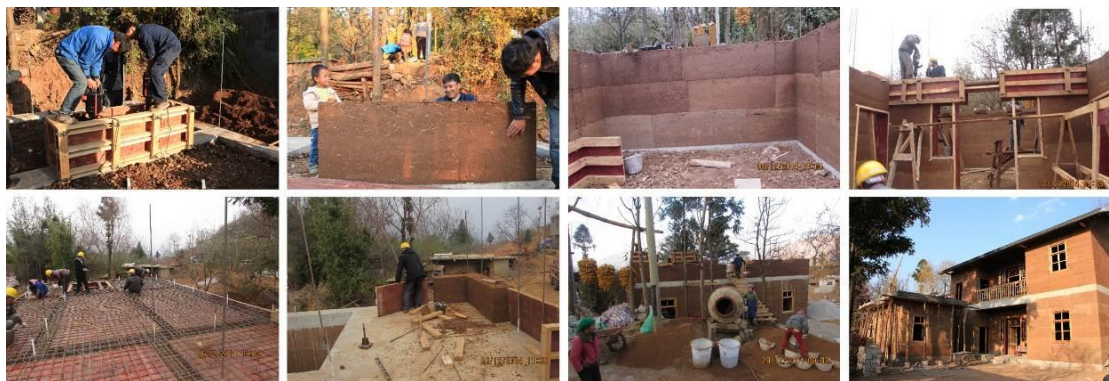
Figure 3- 10. Main structure construction
