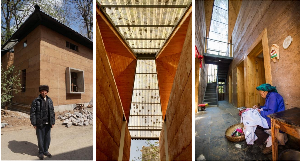
Figure 13-19. Second demonstration rammed-earth building
