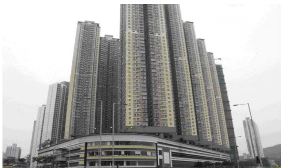
Figure 5: A typical building morphology in Hong Kong: tower blocks sitting on a podium that occupies the entire site. When podiums are very close together, they significantly reduce the air space at pedestrian levels.
