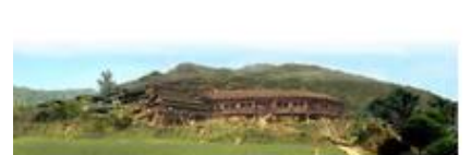
Post-earthquake Reconstruction Project Ma'anqiao Village, Sichuan (2008-2011)
